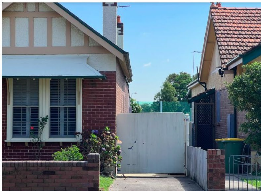
Figure 19 – View of front driveway and neighbouring dwelling , gate to be replaced, view looking northwest (Source: 3+1 Heritage, 2023)
