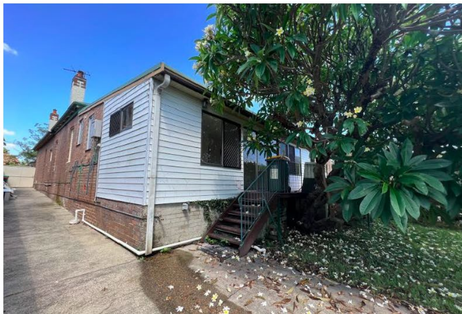
Figure 23 – View of the rear of the dwelling, with timber deck to be replaced and tree to be removed, view looking south (Source: 3+1 Heritage, 2023)
