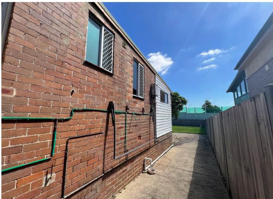
Figure 21 – View of the rear of the dwelling with weatherboard extension, looking towards rear garden, northwest (Source: 3+1 Heritage, 2023)
