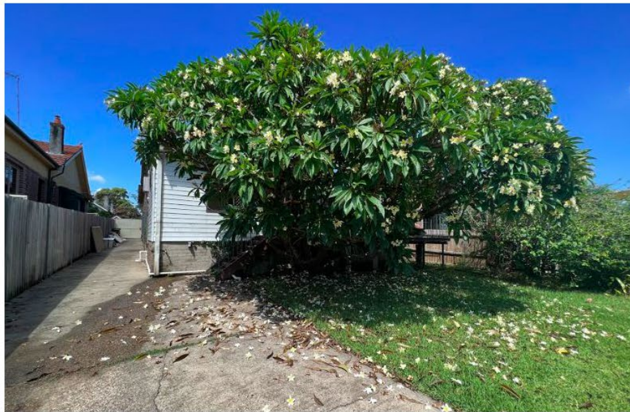
Figure 26 – View towards rear of the dwelling and driveway, view looking southeast (Source: 3+1 Heritage, 2023)
