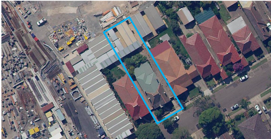
Figure 16 – Aerial view of site April 2018 showing construction site for arterial road and impact on the garden of the subject site (Source: SIX Maps)
