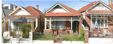
11-15 Macaulay Road, Stanmore Verandah fretwork Casement Windows Palisade front fence
