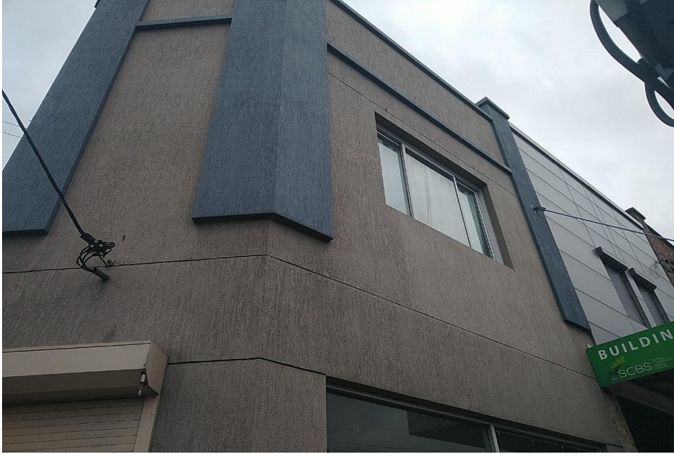
Photograph 3: Level 2 of 612 Parramatta Road - looking north west
