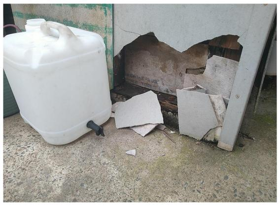
Photo 8: Potential asbestos containing materials at rear of property
