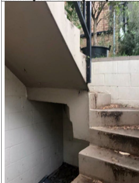
Stair up from entry – view east
