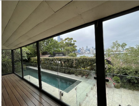
Figure 9 – Standing view from covered rear terrace (photo supplied by applicant)
