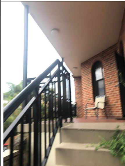
Stair up from entry – view west
