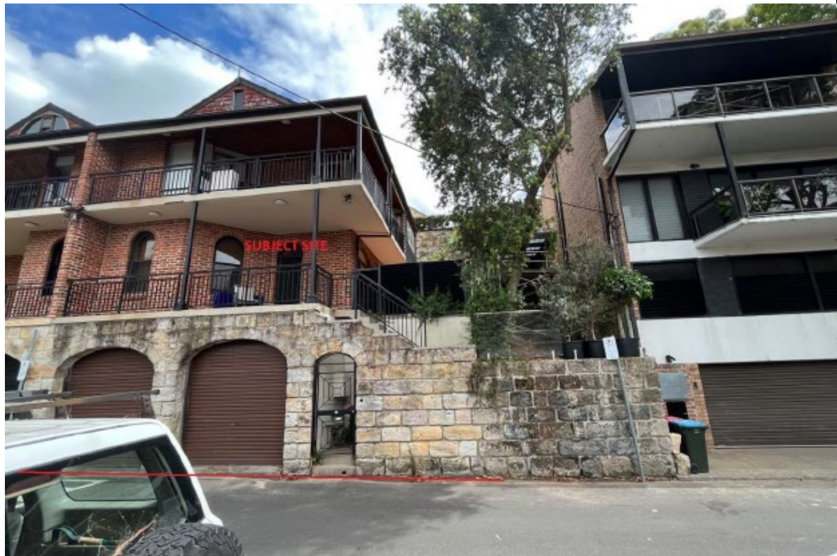
Figure 4 – Streetscape view of subject site, northern aspect
