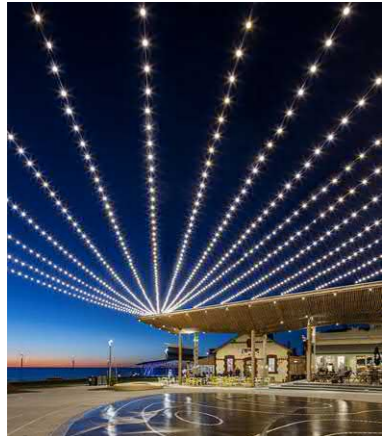
(A) Catenary Feature Lighting
