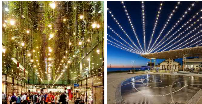
Catenary lighting elements
