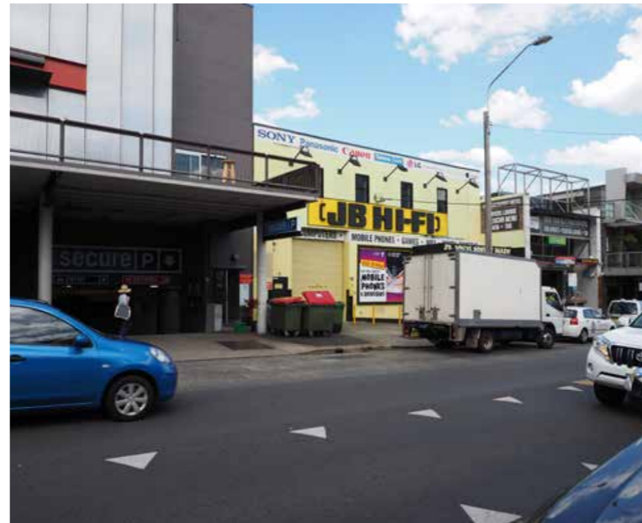
The eastern edge of Norton Street is characterised by large blocks, poor built form and low footpath amenity with many driveway entries.
