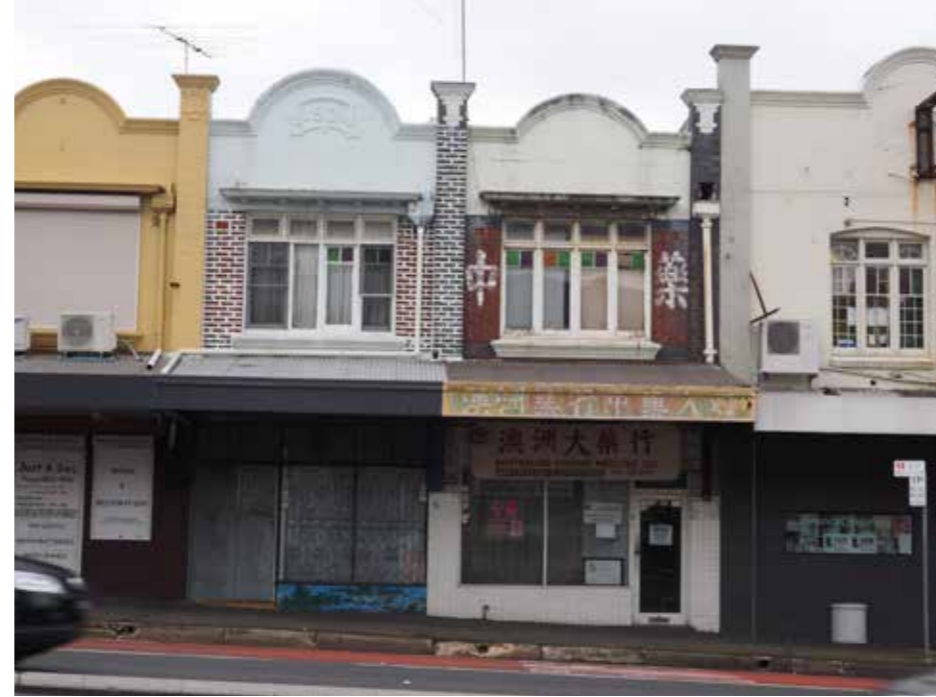
Declining retail development along Parramatta Road needs revitalisation.
