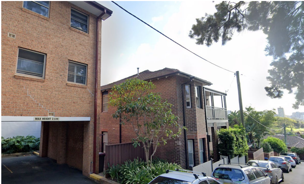
View of No. 2-4 Clifton Street and No. 6 Clifton Street
