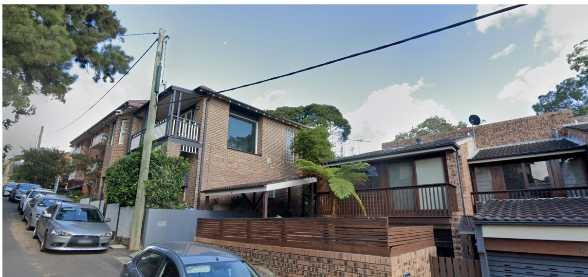
View of No. 6 Clifton Street and No. 8-10 Clifton Street
