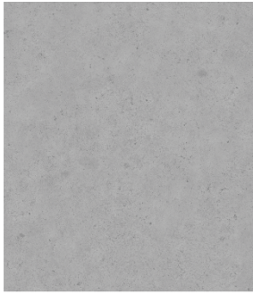
Front Fence Off Form Concrete
