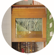
TIMBER FRAMED JOISTS AND WINDOWS
