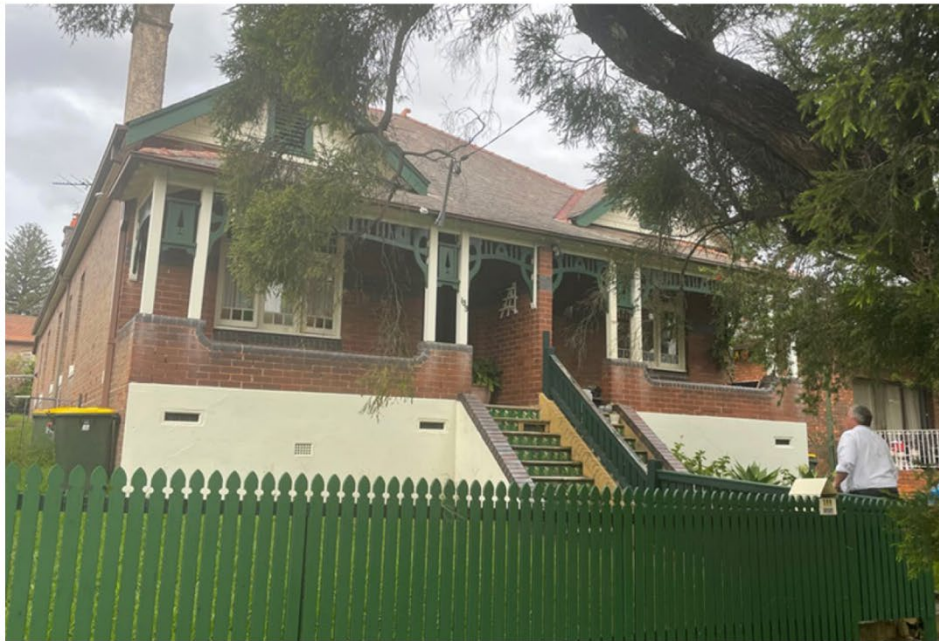
Photo 1: 199 to 197 Alt Street semi-attached dwellings 199-199 Alt Street, Site Visit 22/02/2023
