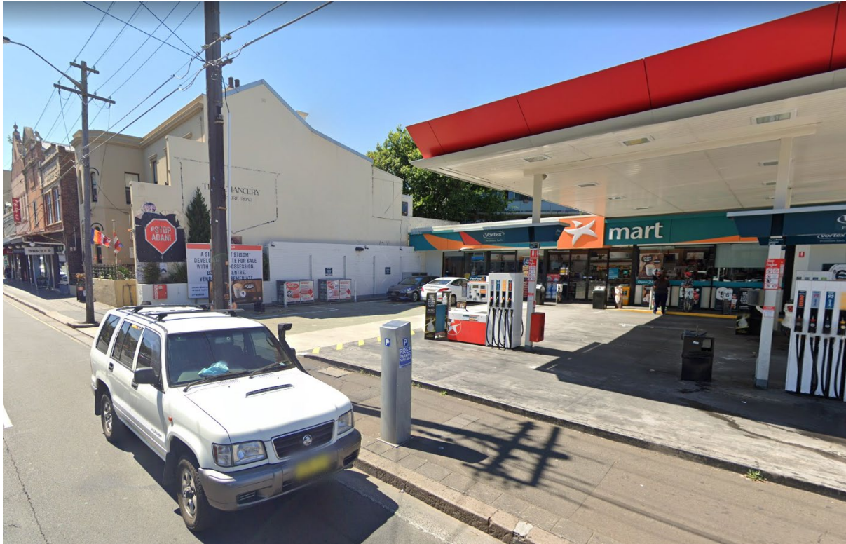
Images of 26-26 Enmore Road prior to demolition in late 2021
