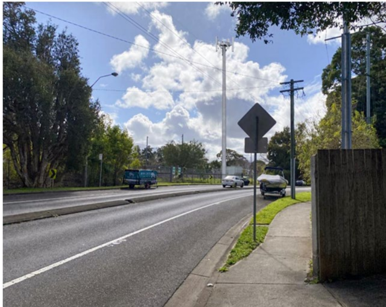
Figure 3 - View 3 of the proposed facility looking south from the northern entry to 130 William Street
