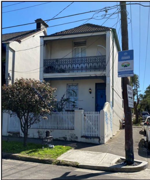
Figure 2: View of subject site from Lynch Avenue
