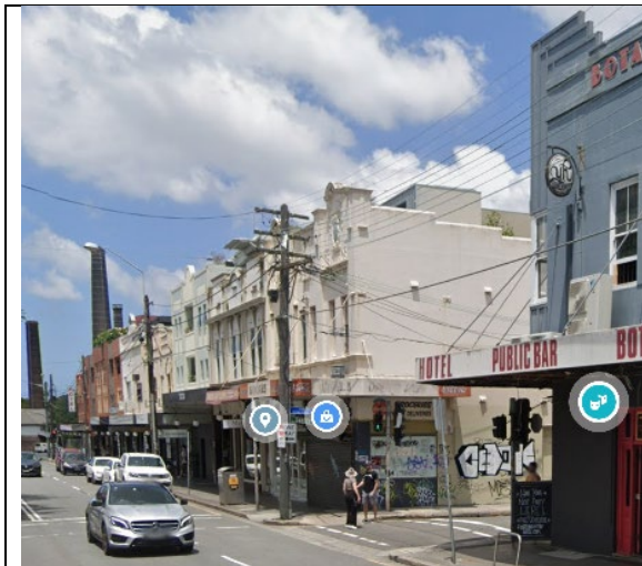
Figure 7: View at four storey development at 601-603 King Street. Source: google maps
