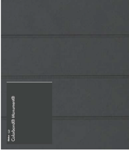
Granny Flat First Floor Walls - FC Cladding Boral Scyon Axon Smooth 133 Dulux Colorbond® - Monument
