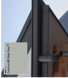
Fascia, Gutters & Down Pipes - Steel Dulux Colorbond® - Shale Grey
