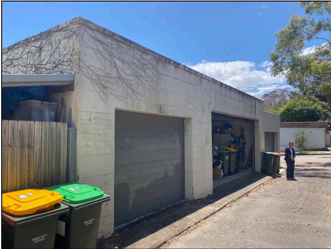
Figure 5: View of existing structure from Brighton Lane
