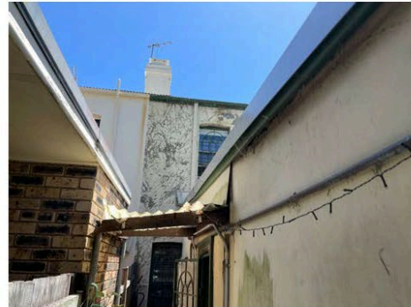
Figure 9: View of ground floor side passageway.
