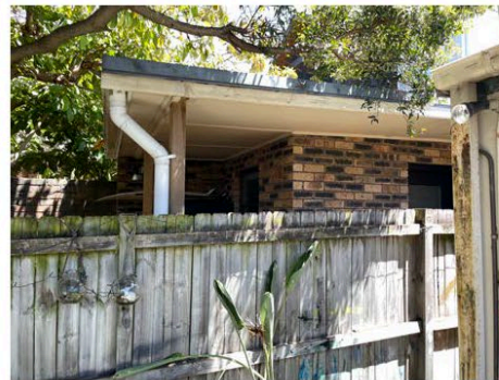
Figure 12: View of the rear of No.172.
