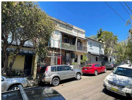
Figure 2: View from Denison Street.
