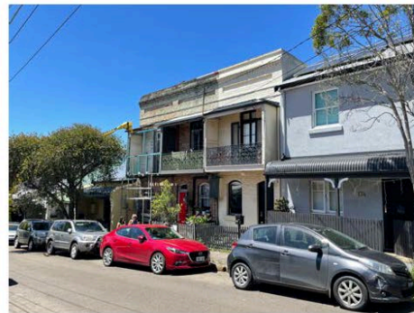
Figure 3: View from Denison Street.
