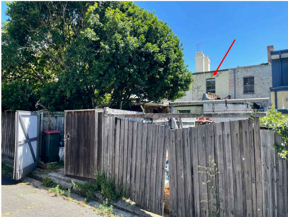
Figure 13: View of the rear elevation from Brooks Lane.
