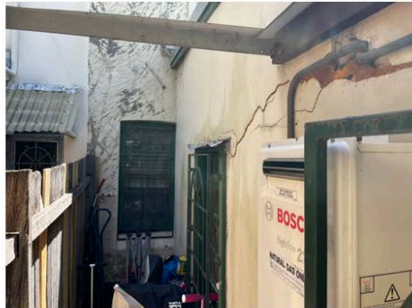
Figure 8: View of ground floor side passageway.
