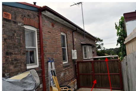
33. Southern side of house. Extg. gates & carport.
