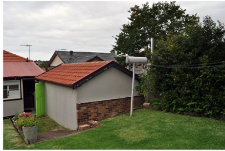
25. Rear of garage.
