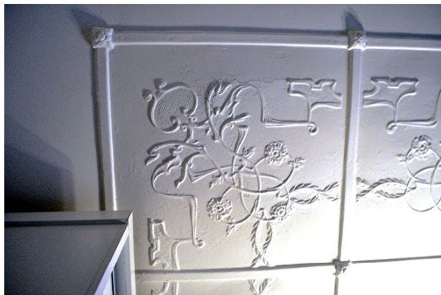
21. Moulded fibrous plaster ceiling- rear bedroom
