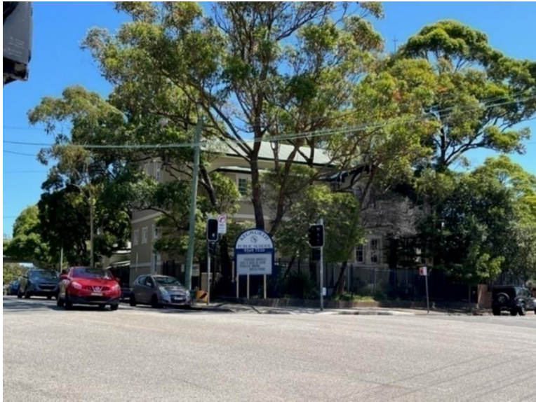
Figure 1112: School looking west from Lords Road/Flood Street
