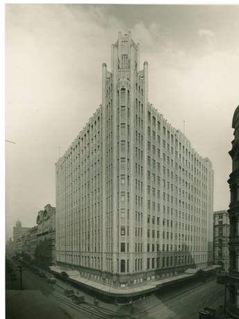
Grace Building, Sydney. Photo by EA Bradford c1930. Museum of Arts & Applied Sciences
