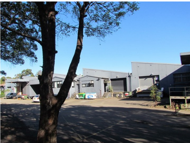
East facades of original factory building have been altered and added to.
