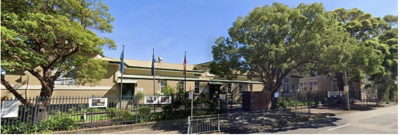
Original 1887 building and primary frontage of the Kegworth Public School to Tebbutt Street.
