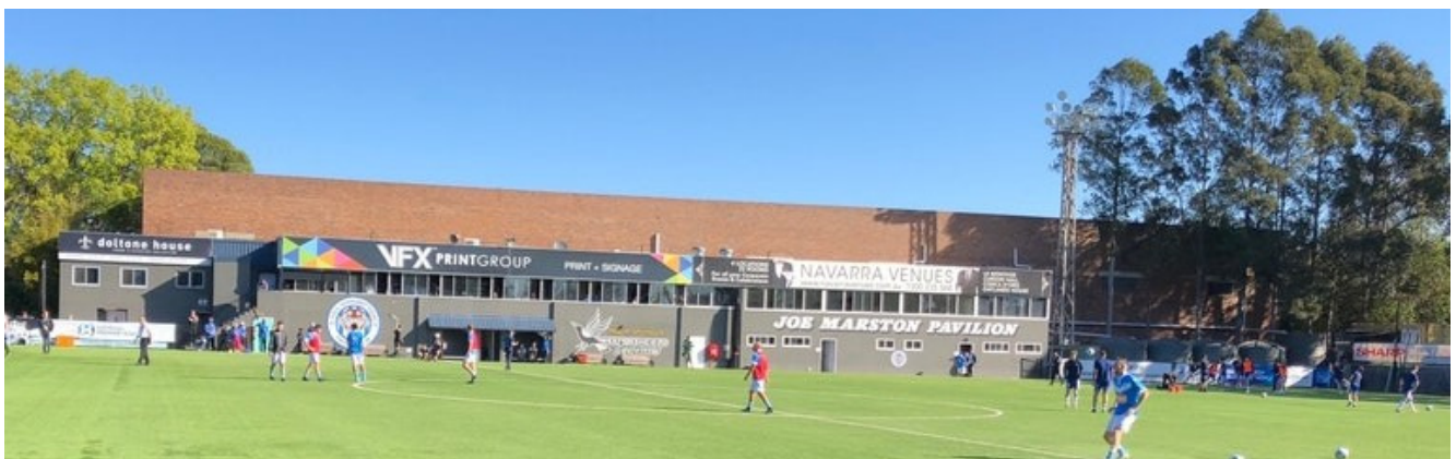
Lambert Park playing field, looking south towards the subject site. Brick parapet wall, seen behind the clubrooms and amenities building, is to be removed in the new development
