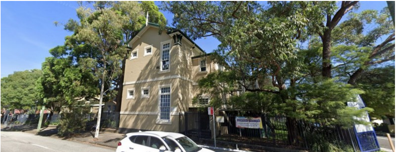
Kegworth Public School, viewed from the corner of Tebbutt Street and Lords Road, with the 1896 Infants Block in the foreground
