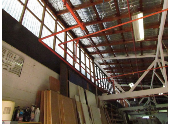
Polycarbonate clerestory and exposed roof framing in the rear unit
