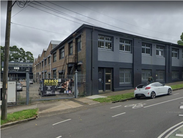
67-75 Lords Road street frontage , viewed from SW corner of the site
