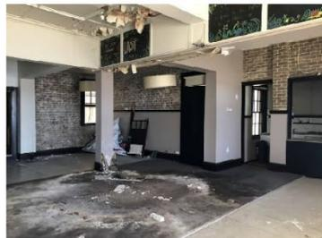
Figure 23: Ground floor room showing deterioration of paint, damage to carpet over terrazzo.
