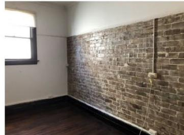
Figure 32: First floor room showing facebrick and plaster wall finishes.
