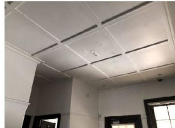
Figure 30: Ceiling to stair landing showing flaking paint.
