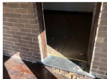
Figure 26: Damaged slate threshold.
