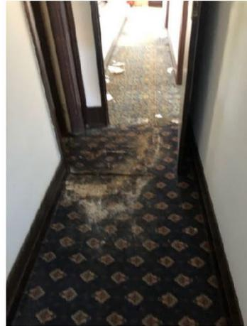
Figure 40: Eastern hallway on first floor showing poor condition of carpet.
