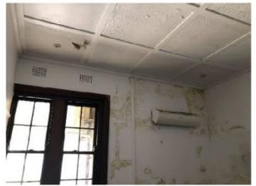
Figure 38: Room next to first floor bathroom, facing north, showing severe water damage to wall and ceiling.
