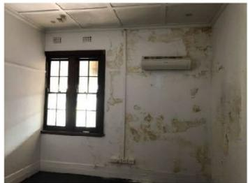
Figure 37: Room next to first floor bathroom, facing north, showing severe water damage.
