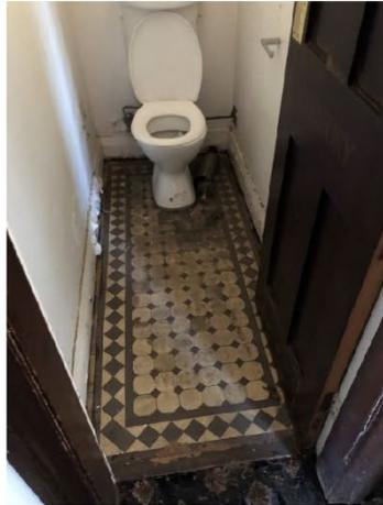
Figure 39: First floor bathroom showing tessellated tiles, skirting and walls, in poor condition.
