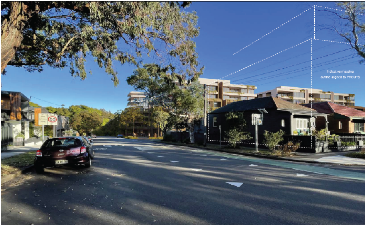
Figure 15: Detailed view along Lords Road looking west
