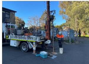
View of monitoring well BH2/GW2 Looking South Inspected 15.06.2022
