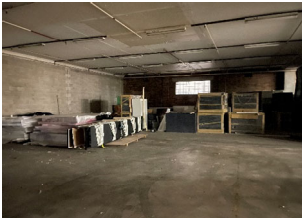
View of inside the warehouse Inspected 15.06.2022
