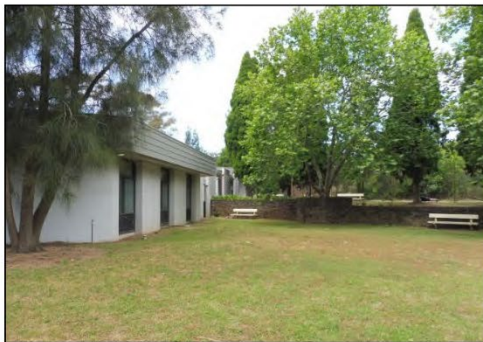
Figure 3.16 The open lawn and terrace retaining wall adjacent to the path extending from the Glover Street entry and B103.
