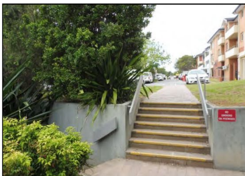
Figure 3.28 The courtyard and steps lead to the existing car parking area and vehicular access to the site. A solid retaining wall also extends between the two levels.
