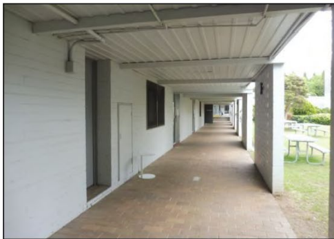
Figure 3.22 Covered wide walkway along the inward facing façade.
