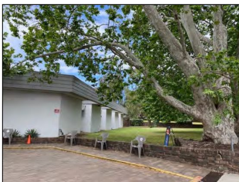
Figure 3.8 The driveway discharges onto Glover Street and is bounded by terraced lawns. The Glover Street end of the driveway is bounded by a low brick retaining wall.
