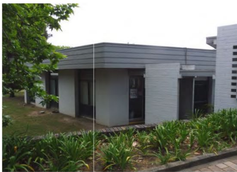
Figure 3.15 B103 is also a single storey painted masonry building that comprises of three wings arranged about a central hexagonal shaped wing. The wings step down and follow the grade of the site.
