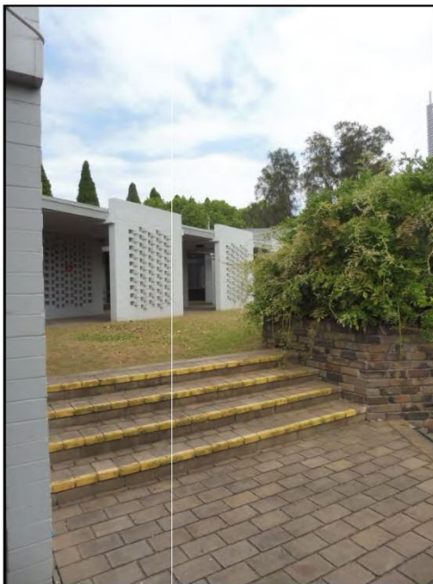
Figure 3.21 The stair wraps around a hexagonal planter.
