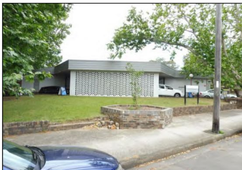
Figure 3.7 B101 which is located close to the corner of Glover and Church Street. A driveway cuts across the corner of the site and extends through a porte cochere that extends along the north western façade and building entry.
