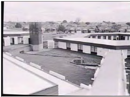
Figure 2.4 Broughton Hall Psychiatric Clinic shortly after completion.
