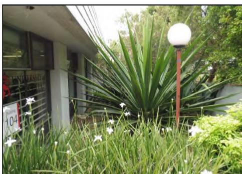
Figure 3.29 Garden beds and planting between the B104 and car parking area. A new suspended ramp and landscaping are proposed in this location.
