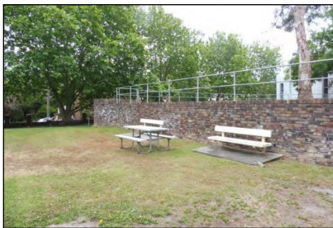
Figure 3.24 Open grassed area and retaining wall between B101 and B105. The wall is topped by a simple pipe steel handrail. A new access ramp (Ramp 2) is proposed in this area and will largely run parallel to the brick wall.
