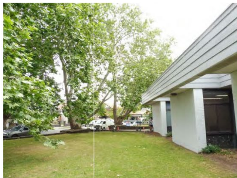
Figure 3.10 The lawn and open areas adjacent to the driveway and western facade of B101 (at left).
