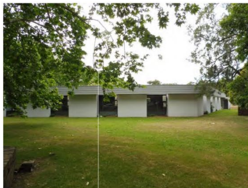
Figure 3.11 B101 is a single storey masonry building with deep fascia and flat roof.
