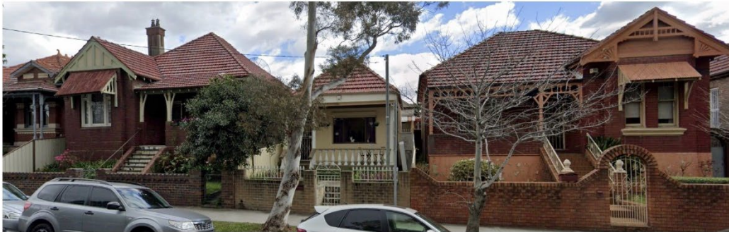
Nos 58-64 to the west side of Percival Road. The diminutive dwelling on the subject site is to the centre.
