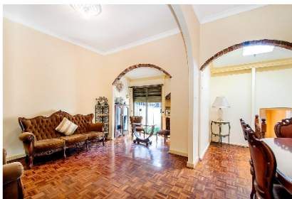
Lounge & Dining Room looking through to the Study and front of the house. No period detail of note remains. Original doors, windows, linings, decorative trims, etc have all been removed.
