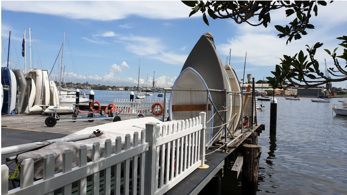
View of the existing skid and existing pier
