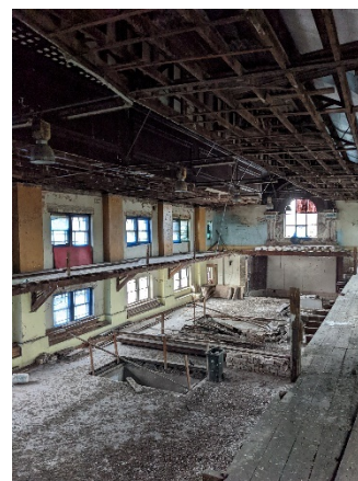
Existing condition of the upper floors
