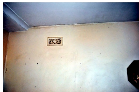
29. Plaster vent, ceiling modifications.
