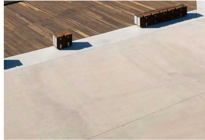
Insitu concrete paving
