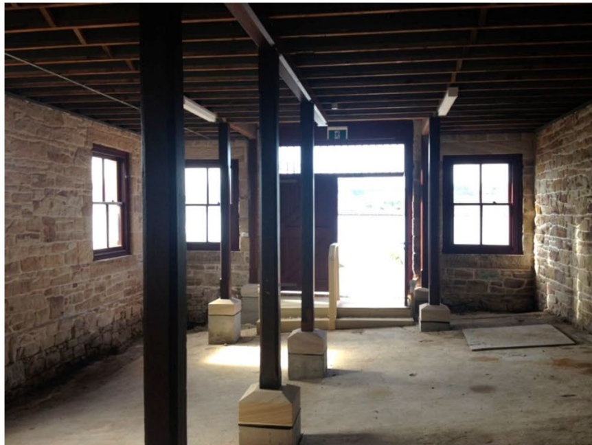
Figure 7: Ground floor of Fenwick's Stone Building looking east towards building entrance. Note the steep slope of the floor.
