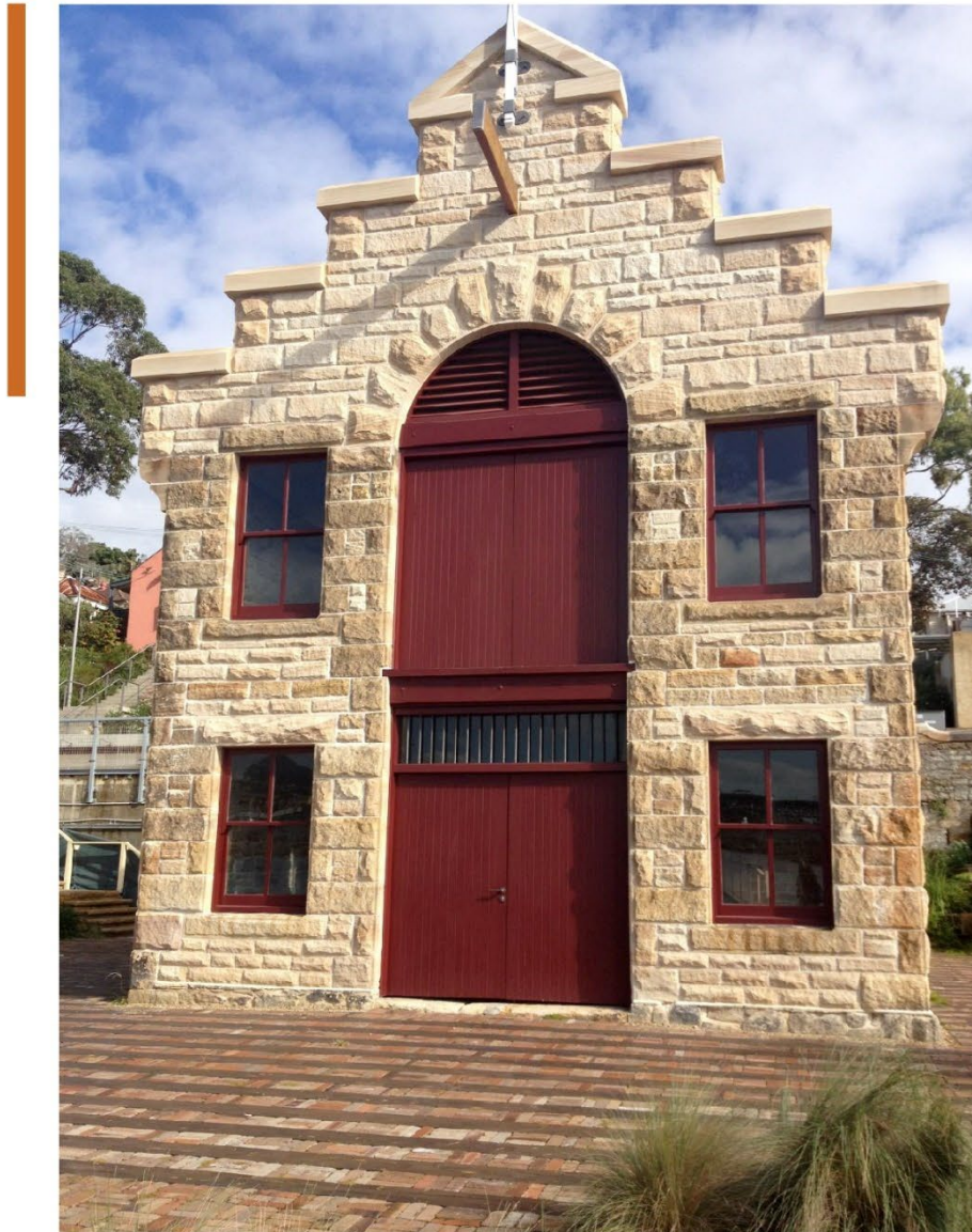
Figure 3: Image showing the front (eastern) elevation of Fenwick's Stone Building. Note the parapeted gable which has been recently restored/reinstated and other sandstone blocks which appear to have been replaced.
