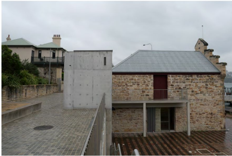
Figure 20: View of the southern elevation of the Fenwick's stone building showing new concrete lift and concrete walkway along the southern side of the building, constructed in 2015. The paved area at right next to the southern elevation is the area proposed for outdoor seating, umbrellas and coffee cart.
