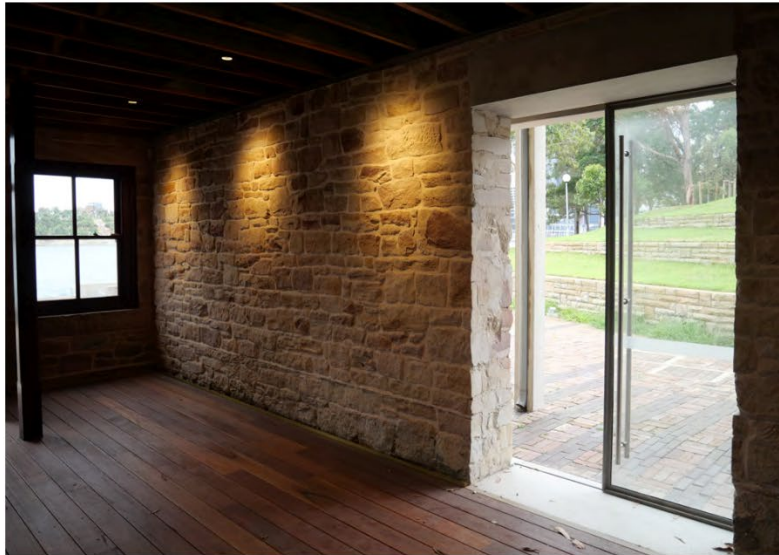
Figure 30: Detail view of the modern opening cut through the sandstone walls to the southern elevation.
