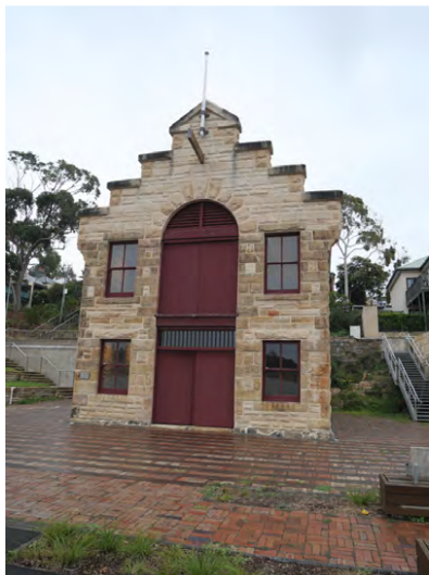
Figure 13: View of the east elevation of the Fenwick's stone building, with the stepped parapet reconstructed in 2011.
