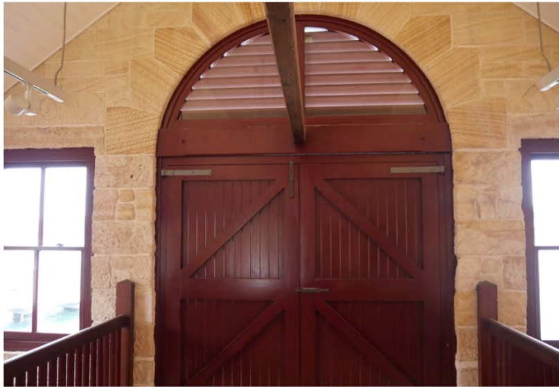
Figure 38: View of the timber double doors to the first floor void and arched vent over.
