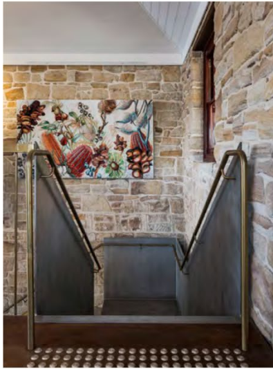
Figure 46: View of the contemporary steel stair from the first floor down to the ground floor.
