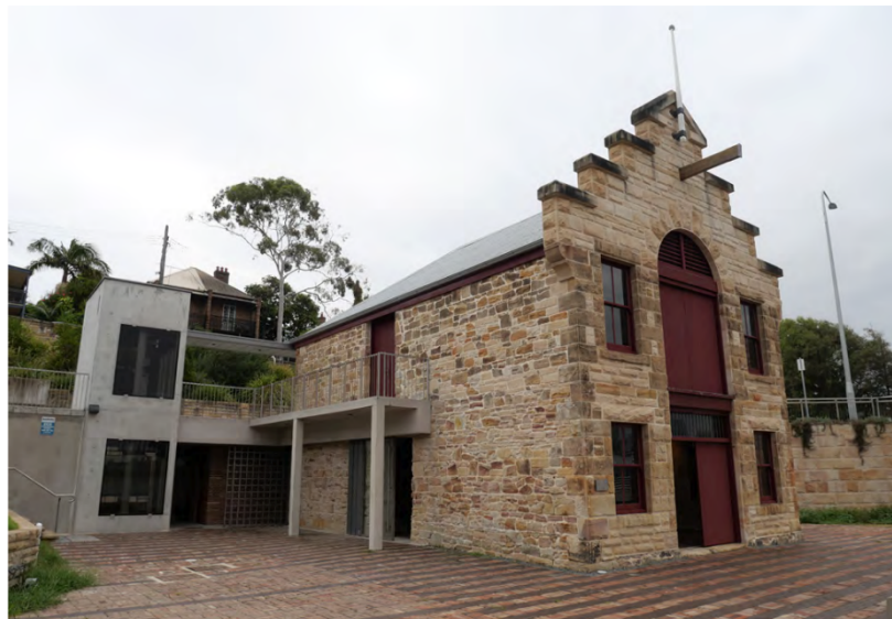
Figure 6: View of the south-eastern corner of Fenwick's stone building. Note the modern concrete lift and elevated concrete walkway to the southern elevation, constructed in 2015.
