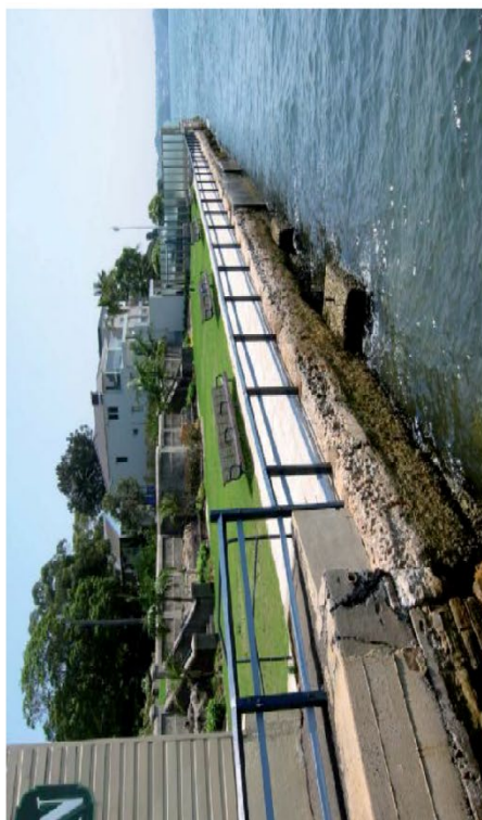
Above: Existing seawall on Thornton Park. Frontage has been recently repaired. The type of repair is unsympathetic to the heritage significance of the seawall and should not be replicated at the 2 - 8 Weston Street site.
