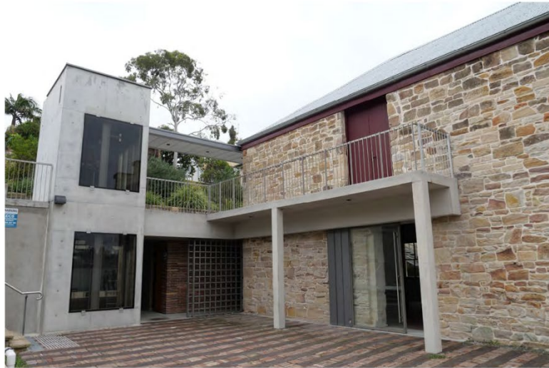
Figure 22: View of the southern side of Fenwick's stone building showing new concrete lift and concrete walkway along the southern side of the building constructed in 2015. The paved area in foreground is the area proposed for the outdoor seating.
