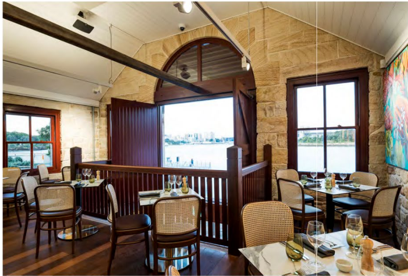
Figure 36: View of the void and timber balustrade to the eastern door openings. A new semi-frameless glass enclosure is proposed to the existing void space. The existing timber balustrade is to be retained.
