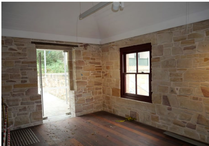
Figure 43: View the new door opening to the western elevation of the first floor.
