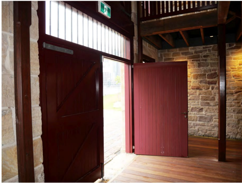
Figure 28: View of the ground floor east elevation doors. A new semi-frameless glass enclosure is proposed to the existing void space to allow the existing solid doors to be open during operating hours but still provide weather protection for visitors.
