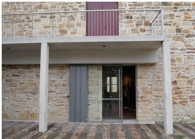
Figure 23: View of the new southern ground floor entry to Fenwick's stone building constructed in 2015 showing new concrete walkway along the southern side of the building. This new entry point was constructed to provide level disabled access from the reserve. This doorway will be used to service the outdoor seating area proposed.
