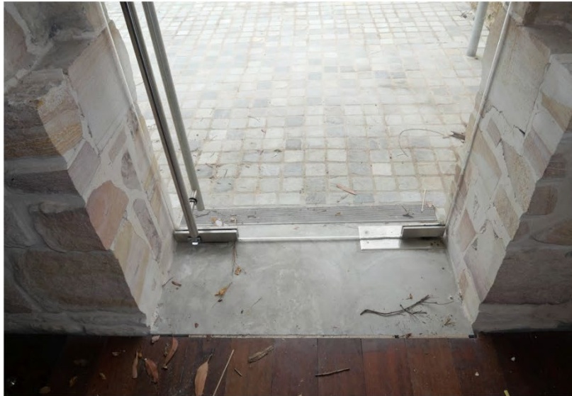
Figure 44: View of the new door opening and concrete threshold on the first floor western elevation.
