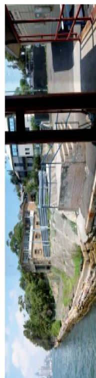
Above: Existing seawall on Thornton Park. Frontage has been recently repaired. The type of repair is unsympathetic to the heritage significance of the seawall and should not be replicated at the 2 - 8 Weston Street site.
