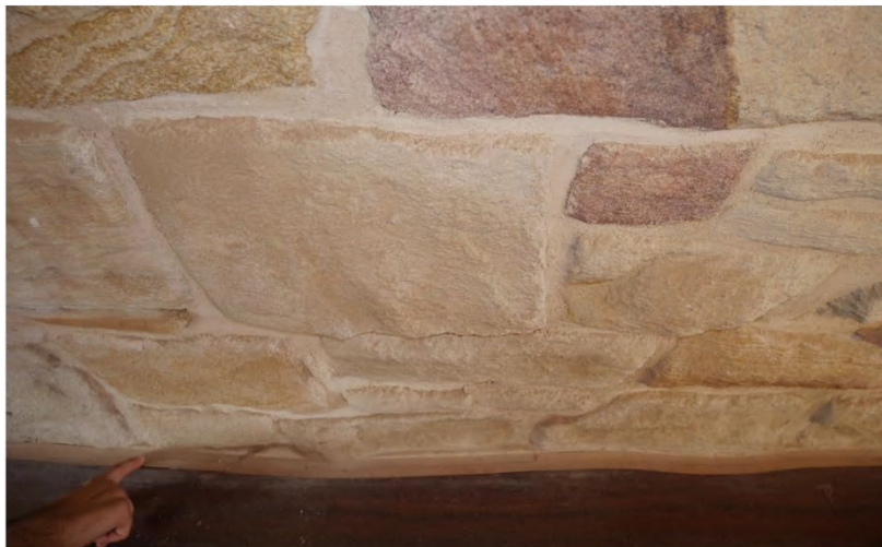
Figure 45: View the flexible sealing between the timber floors and sandstone walls.
