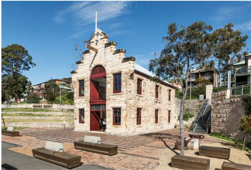
Figure 7: View of the north-eastern corner of Fenwick's stone building. The stepped parapet was reconstructed in 2011.
