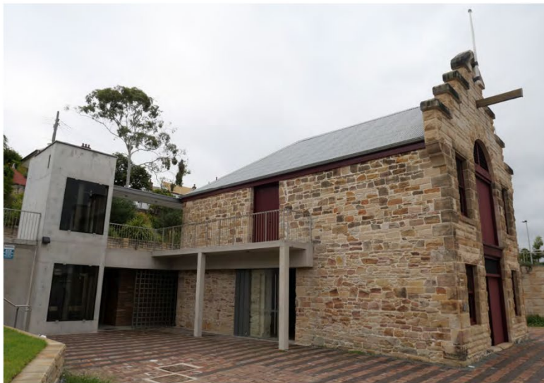
Figure 21: View of the south-eastern corner Fenwick's stone building showing new concrete lift and concrete walkway along the southern side of the building, constructed in 2015. Note the paved area in centre foreground is the area proposed for outdoor seating, umbrellas and coffee cart, between the southern elevation of the building and the retaining wall at left.
