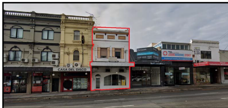
Figure 2: View of the existing building within the Parramatta Road streetscape
