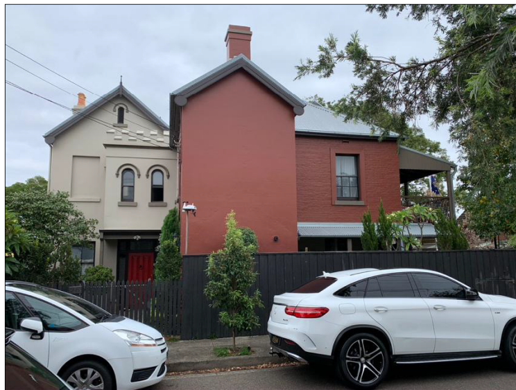
Figure 29: The site from Oxford Street. The area of proposed works is not visible.
