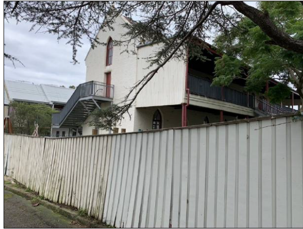
Figure 24: The two storey classroom within Athena School on the corner of Baltic Street and Fitzroy Lane, from Fitzroy Lane.
