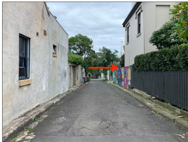
Figure 19: General view west along Fitzroy Lane from Oxford Street. The arrow points to the proposed location of the garage. The southern end of the two storey classroom building at the adjoining Athena School is visible beyond the site.
