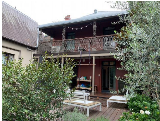
Figure 13: The hipped roof central section of the building with the restored two storey verandah.
