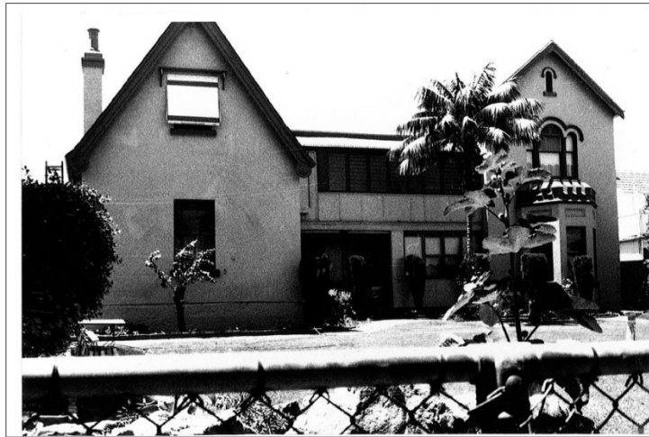
Figure 5: Convent west elevations, c.1960s and 1970s. Good Samaritan Archives, cited in the CP 1998 .
