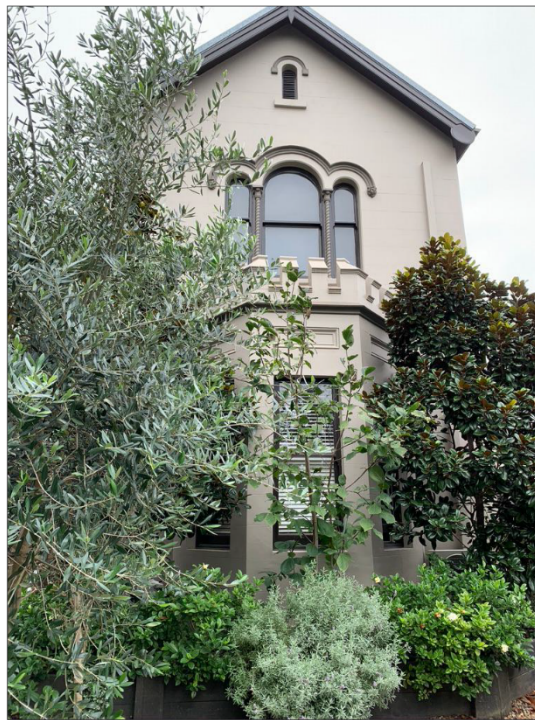
Figure 12: Western elevation of the southern wing of the building. This wing is in the Victorian Italianate Style, with Gothic Style overtones.
