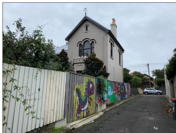
Figure 7: High timber lapped and capped fence along the southern boundary (Fitzroy Lane). Also showing a view towards the site on approach from the south.
