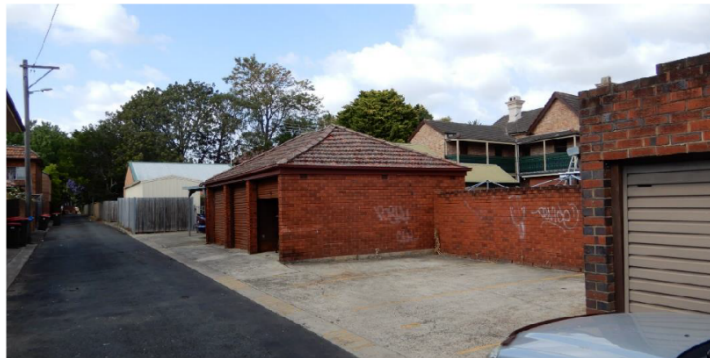
Figure 11: view from near the rear of the subject site looking south-west between garages at the rear of properties facing Victoria Street, looking towards the back verandahs of the Victorian mansion at 118 Victoria Street.
