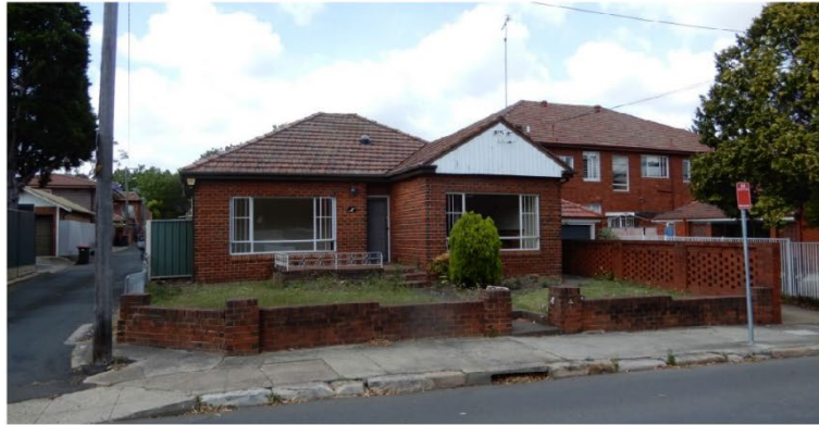
Figure 14: the northern front of the house facing Clissold Street. (Source: NBRSArchitecture 2019):
