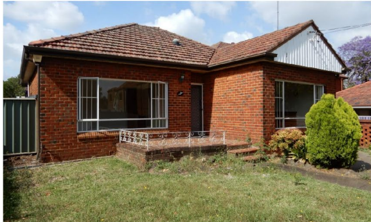
Figure 15: close up of the northern front of the house.
