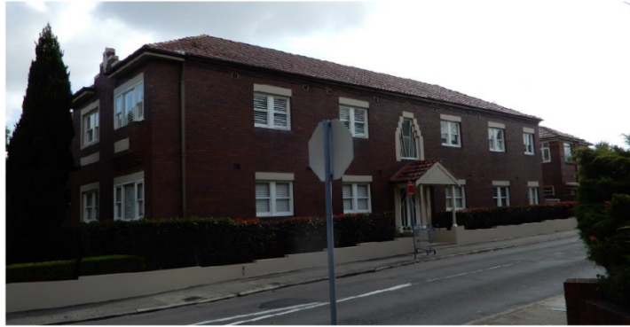
Figure 10: 1930s flats at 114A Victoria Street are opposite the subject site to the north.
