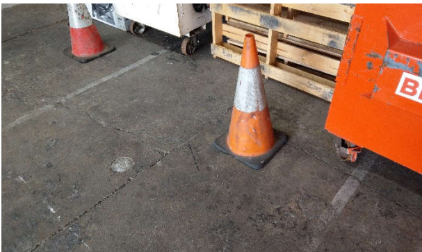
Photographs 15: Identified reinstated concreted core hole location at 206 Parramatta Road which suggests that this area was previously investigated.
