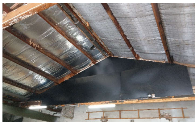
Photograph 12: SMF as sarking insulation beneath the roof observed at 206 Parramatta Road.
