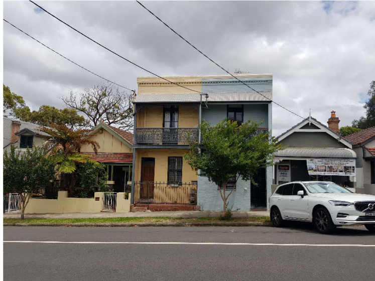
figure – 03 View of the front of 220 from Young Street.
