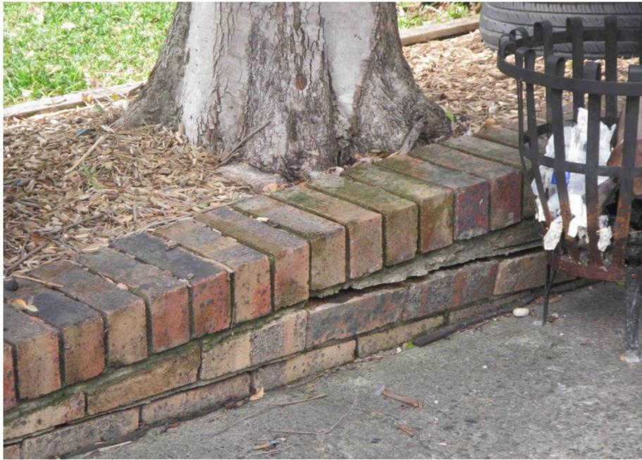
**Figure 10 Shows Tree 6 in close proximity to the existing dwelling and damaging the existing brick retaining wall and driveway area.**
