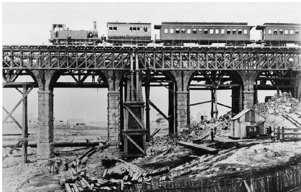
Figure 4: Construction of the Whipple Truss bridge 1886 (Northpoint Heritage: 37)
