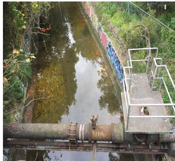
Figure 7: Brick lined Hawthorne Canal at Parramatta Road
