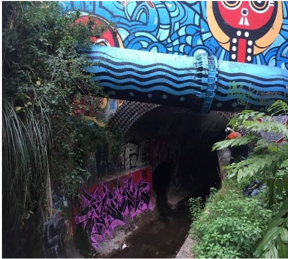
Figure 12: Culvert and Hawthorne Canal running under Longport Street, Lewisham
