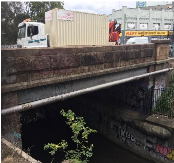
Figure 6: Battle Bridge over Hawthorne Canal Northern side
