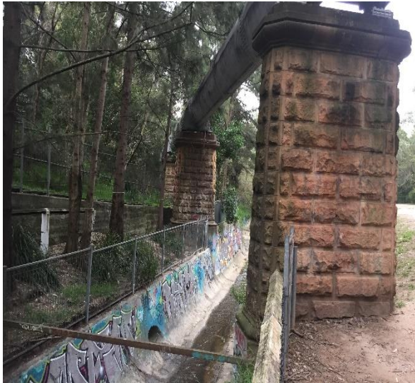
Figure 8: Stone faced supports of the sewage aqueduct in Cadigal Reserve
