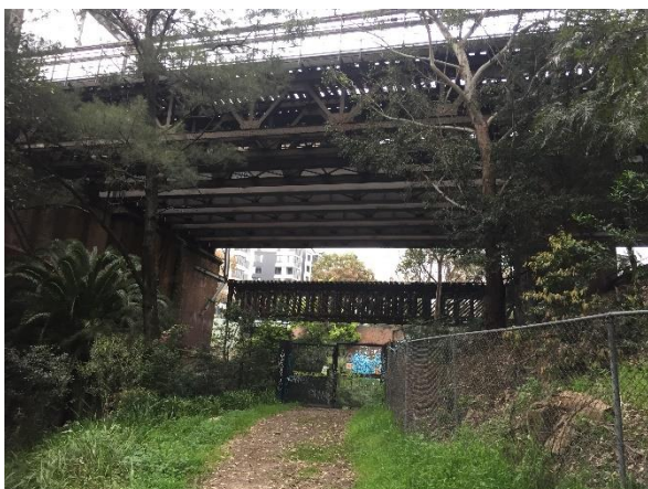
Figure 6: Train infrastructure, Cadigal Park
