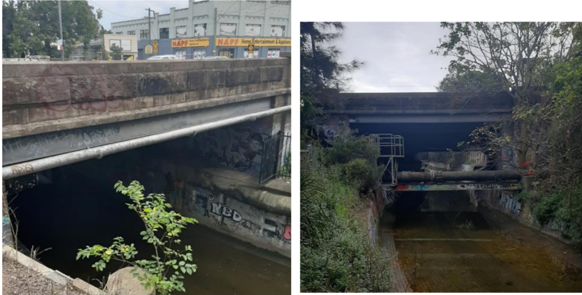
Photo 9: Parramatta Road bridge over Hawthorne Canal containing potential microbat roosting habitat
