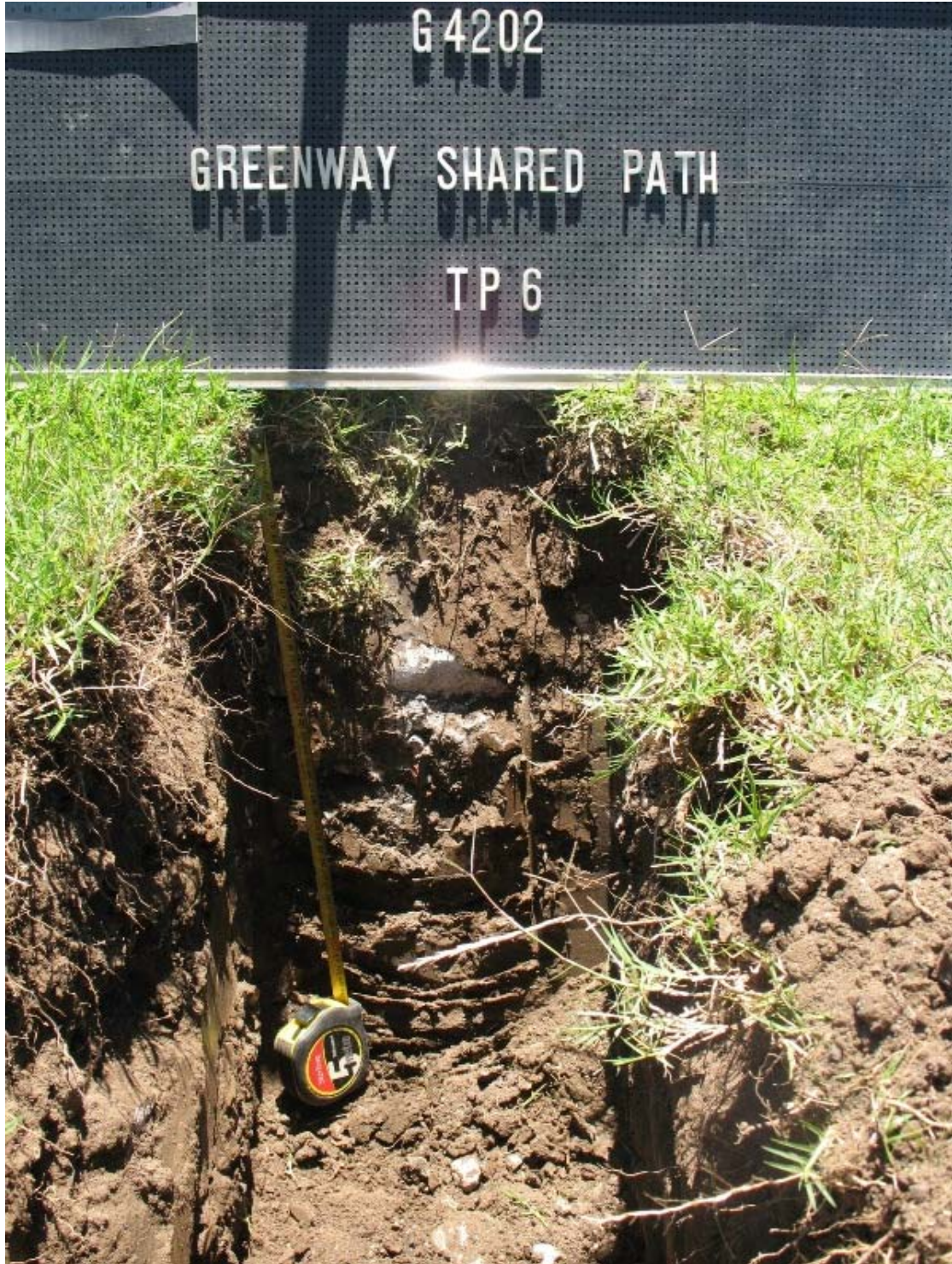
Test Pit 6 (tape extended to 500mmm)
