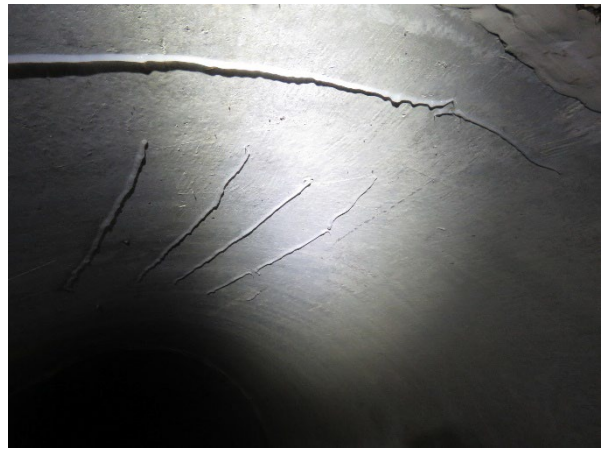
Compensatory silicone habitat installed
