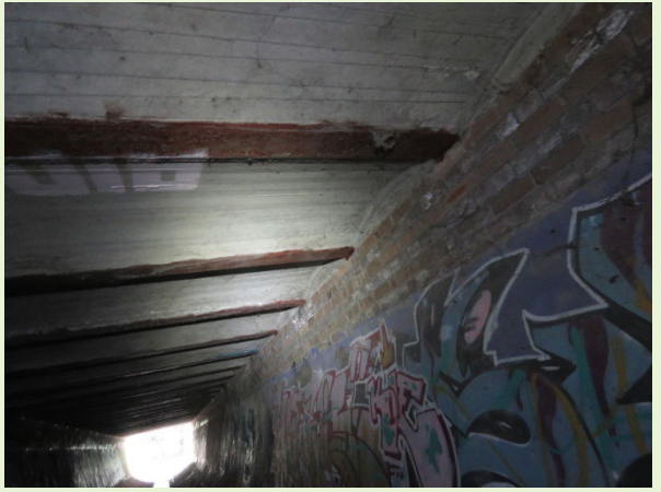
Roof of culvert showing cobwebs and existing potential habitat
