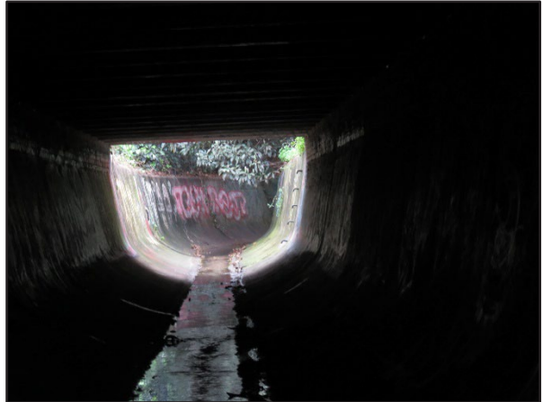
Culvert showing light intrusion
