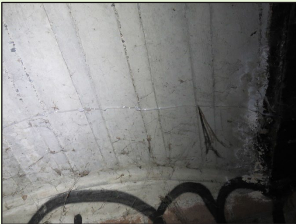
Roof of culvert with compensatory silicone habitat installed.
