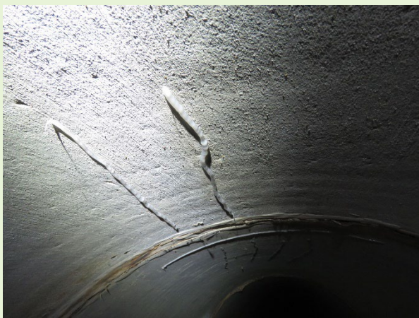
Compensatory silicone habitat installed
