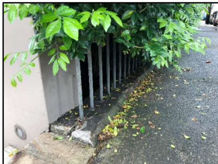
Figure 26. Iron palisade fence and sandstone base to Wharf Road boundary of subject site.
