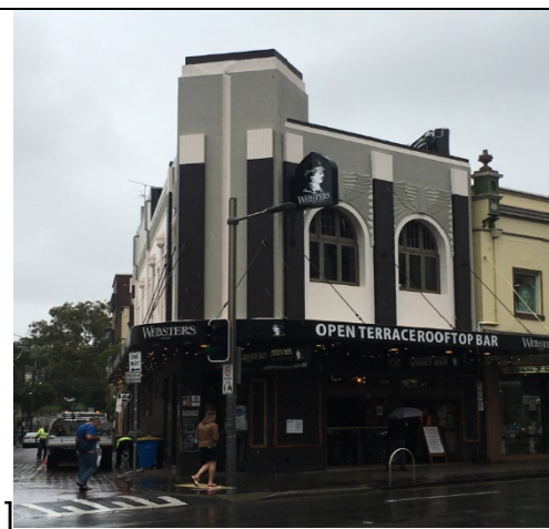
Figure 2: Site photo of existing building taken from King Street.
