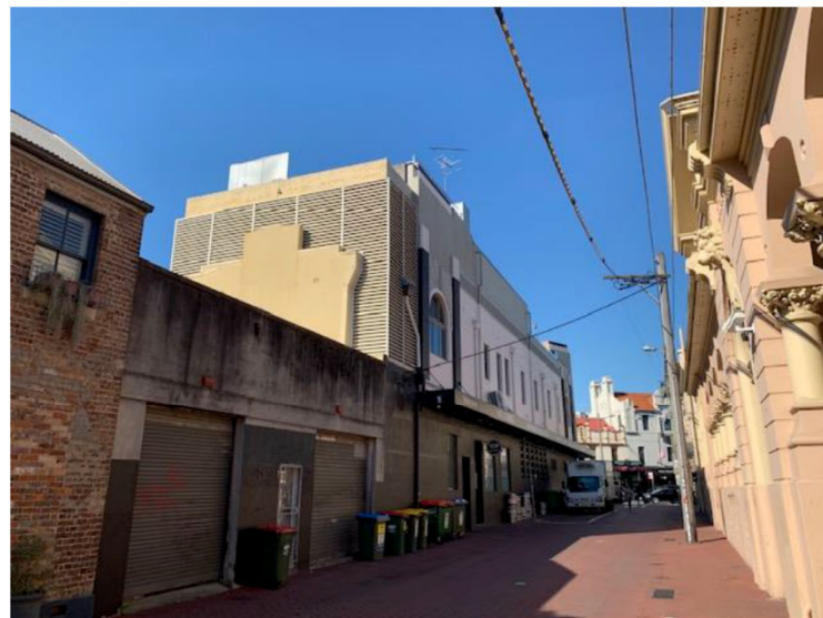
Subject premises from Eliza Street
