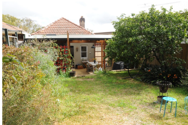
Figure 9: Eastern, elevation of No. 95 Grove Street, Birchgrove from the rear boundary. WPH 2018.
