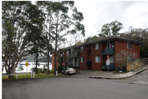
Figure 29: No. 47 Wharf Street, on the Harbour at the corner of Wharf Road and Grove Street. WPH 2018.
