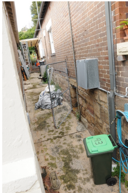
Figure 8: Southern elevation of No. 95 Grove Street, Birchgrove. WPH 2018.
