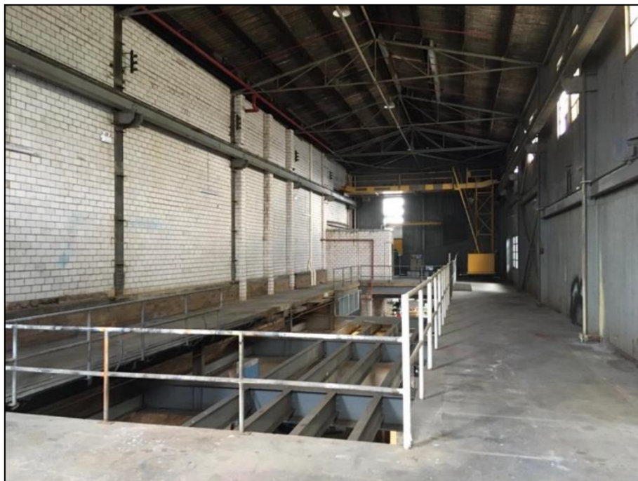
Figure 4: Mezzanine. Note the location of the void makes the space unusable. It would likely have served a particular purpose in relation to the previous industrial use of the site.
