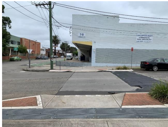
Figure 3.10: Pedestrian Crossing point (Myrtle Street at Carrington Road)
