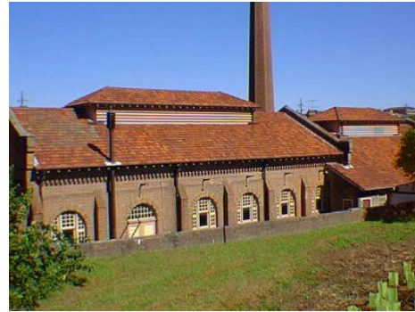
Figure 61: North elevation of pump house with part view of boiler house on left (Source: photograph by James Stephany, image owner Sydney Water, sourced from the NSW Heritage Database 5051444)
