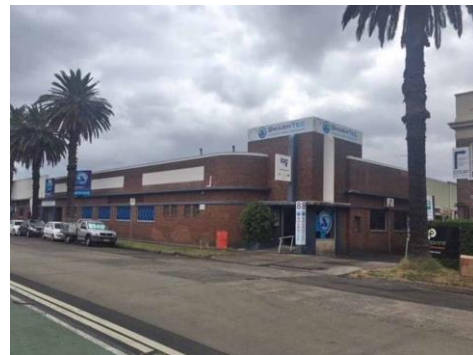
Figure 24: Factory in Inter-War style on Carrington Road. (Source: NBRSARCHITECTURE 2019)
