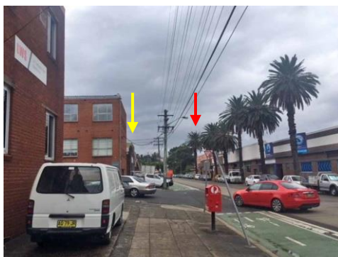
Figure 55: View towards the sewage pumping station from Carrington Road, facing north. The tower of the pumping station is indicated by the red arrow and is obscured by street trees. The yellow arrow shows the approximate location of the subject site, also obscured by trees and buildings.
