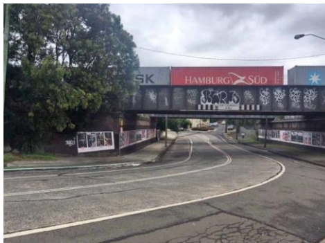
Figure 27: Victoria Road, facing south, showing the railway line. (Source: NBR SARCHITECTURE 2019)
