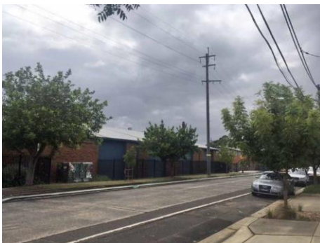
Figure 39: View of 3 Myrtle Street, facing south-east along Myrtle Street. (Source: NBR SARCHITECTURE 2019)
