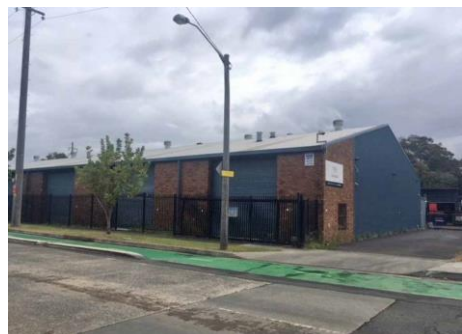
Figure 36: Building at 3 Myrtle Street, showing its frontage to Myrtle Street. (Source: NBR SARCHITECTURE 2019)
