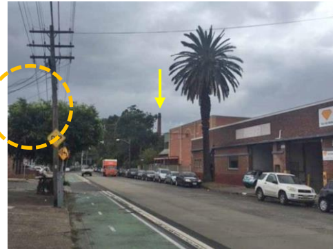
Figure 70: View towards the sewage pumping station from Carrington Road, facing north. The tower of the pumping station is indicated by the yellow arrow, visible at a distance. The proposed development zone (dashed orange) will not interfere with this view of the tower. (Source: NBR SARCHITECTURE 2019)
