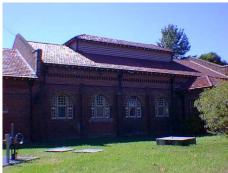
Figure 62: Part south elevation showing pump house (Source: photograph by James Stephany, image owner Sydney Water, sourced from the NSW Heritage Database 5051444)
