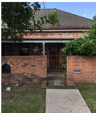
Figure 64: Stone House, including interiors (Source: Marrickville Council, NSW Heritage Database 2030176)
