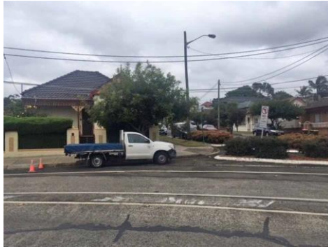
Figure 25: Residential buildings on Myrtle Street, facing south. (Source: NBR SARCHITECTURE 2019)
