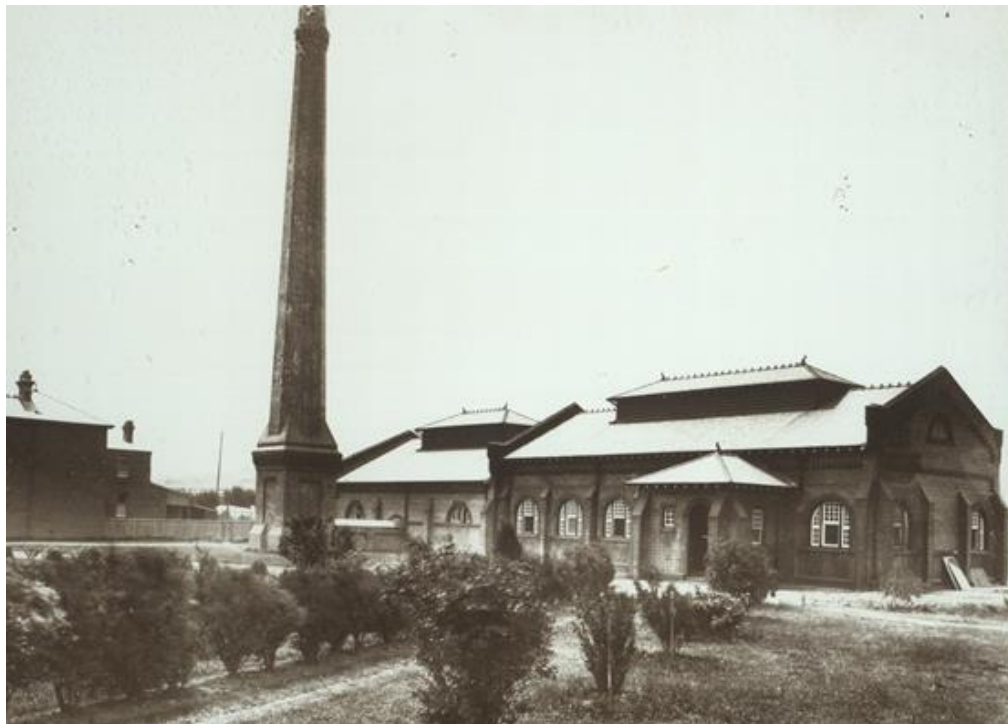
Figure 14: Marrickville Steam Pumping Station - 1897. (Source: Marrickville Council Library and History Services, File LS 2011.008)
