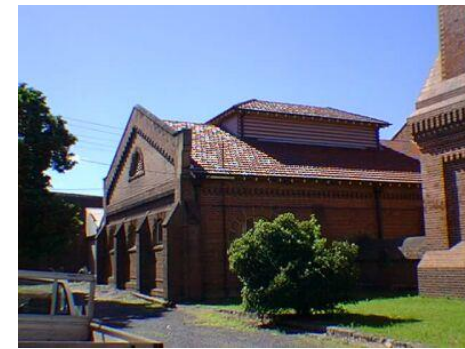
Figure 63: View of west and part south elevation of boiler house (Source: photograph by James Stephany, image owner Sydney Water, sourced from the NSW Heritage Database 5051444)
