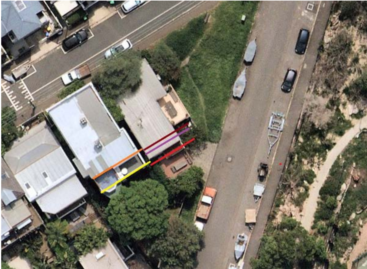
Image 1: Building Location Zone along Short Street
